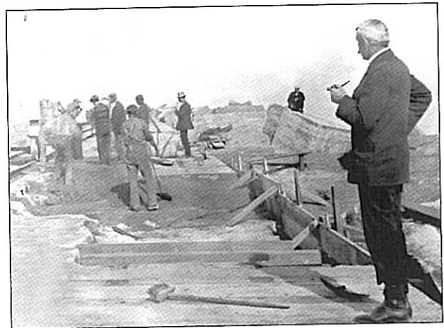
1890's Repairing monoliths on Breakwater after storms
