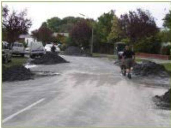
Liquefaction ejecta in piles on road
