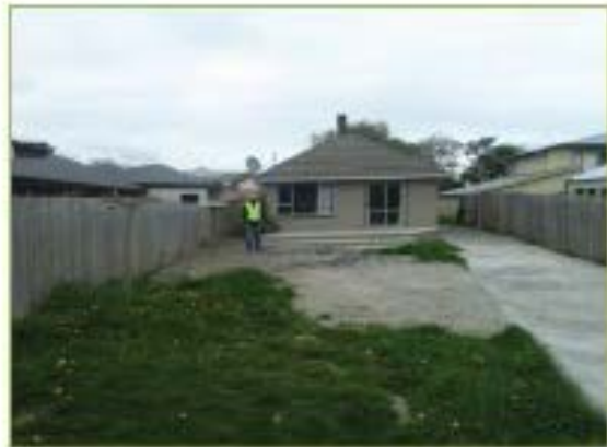
Liquefaction ejecta, dwelling tilting
