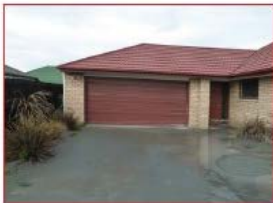
Large amounts of liquefaction ejecta and tilting dwelling
