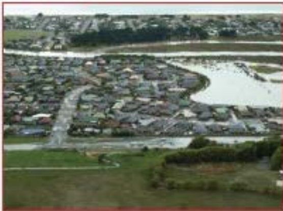
Aerial photo showing liquefaction ejecta on Seabreeze Close
