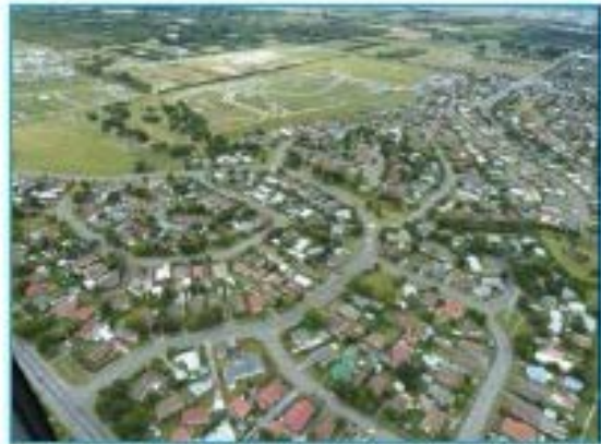
Aerial shot of Broomfield area showing no liquefaction ejecta on the roads or Broomfield Common
