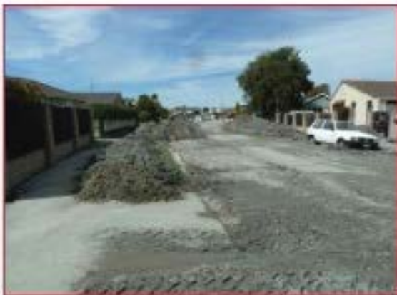
Liquefaction ejecta piles along Androssan Street
