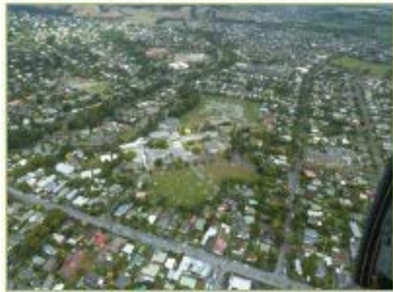
Aerial photo of liquefaction ejecta at Cashmere High School
