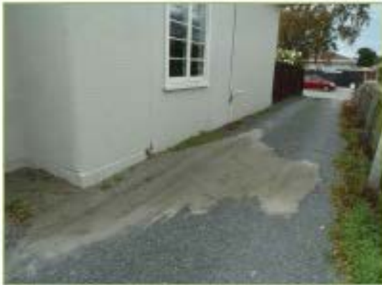
Isolated area of liquefaction ejecta
