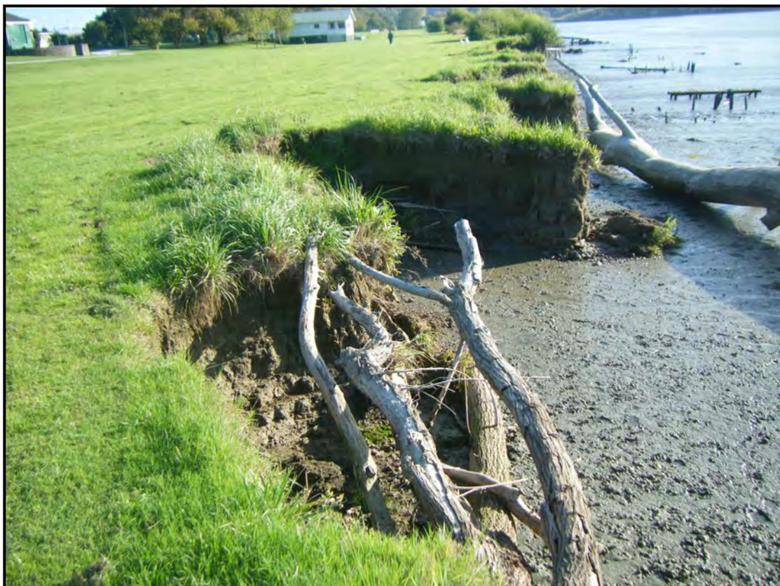
**Photograph 3:** Rotational failures of near vertical river banks along southern end of Kopu Street.
