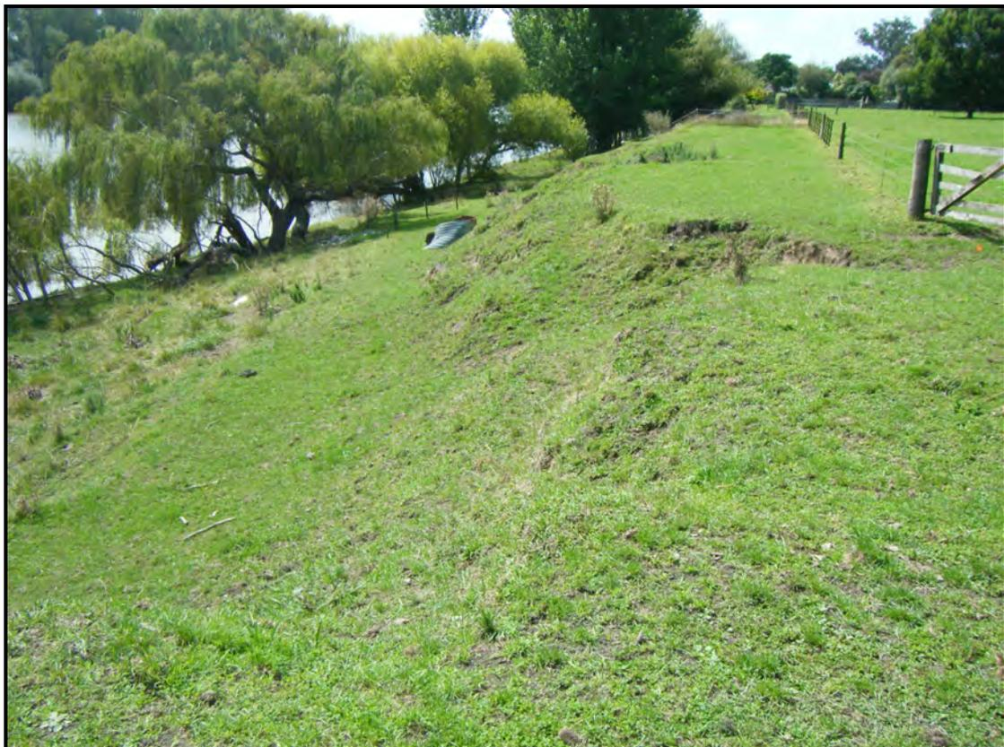
**Photograph 24:** Slope adjacent to SH2 at eastern end (adjacent to Section 4). This instability extends to the west but slope too heavily vegetated to show on photograph and determine extent.
