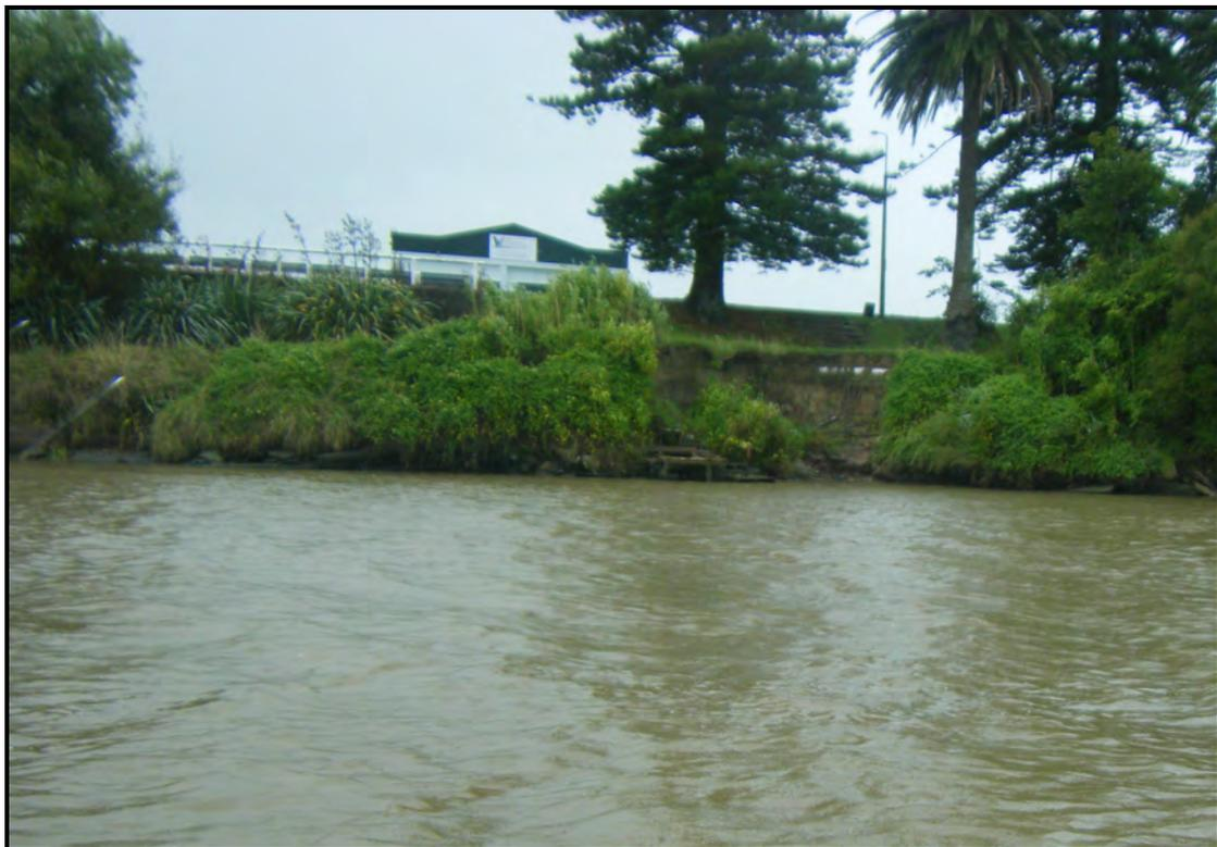
**Photograph 35:** Large rotational failures adjacent to River Parade immediately upstream of SH2 bridge (see also Photograph 37 below).
