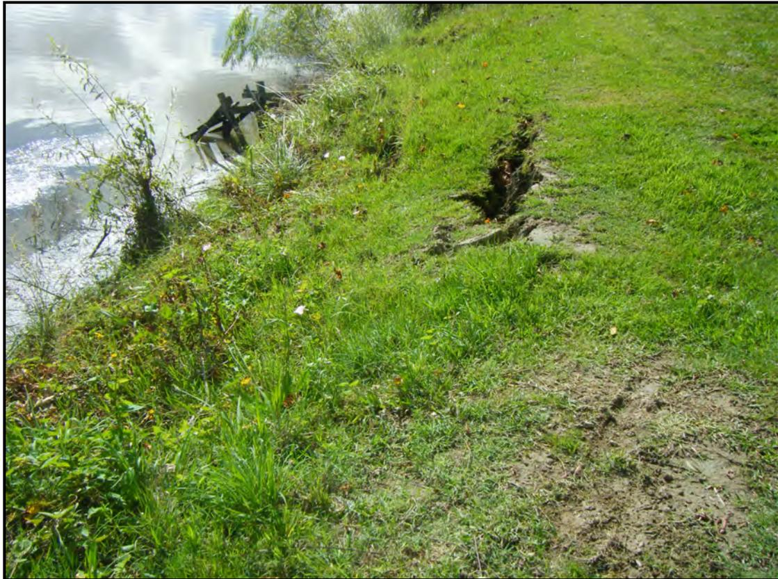
**Photograph 19:** Minor instability of river bank west of SH2 bridge, likely to have been initiated by ongoing scour and loss of toe support.
