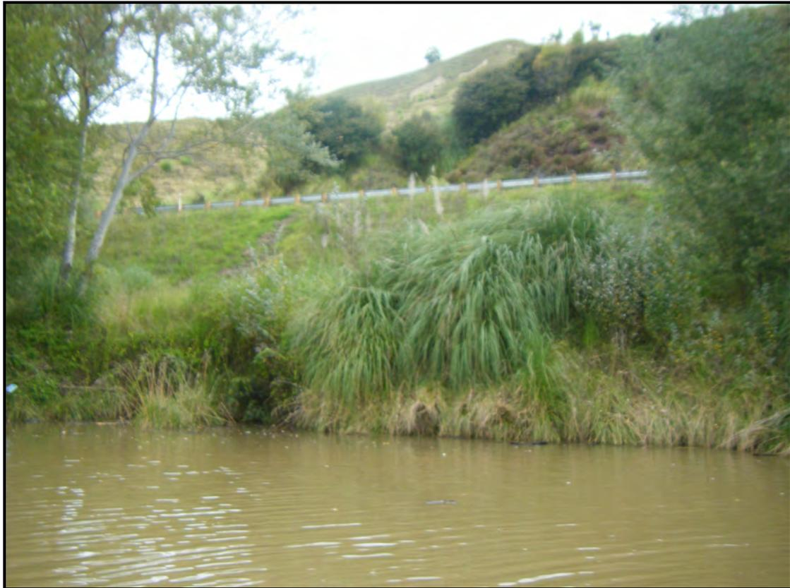
**Photograph 25:** Slope adjacent to SH2 with signs of recent instability and new crash barrier.
