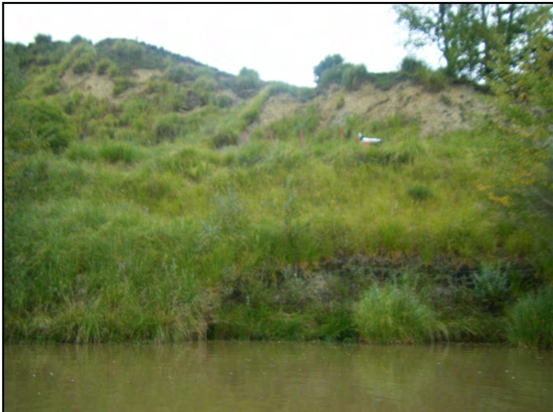
**Photograph 26:** Slope adjacent to SH2 with signs of recent instability of upper slopes and erosion with instability of lower river bank.
