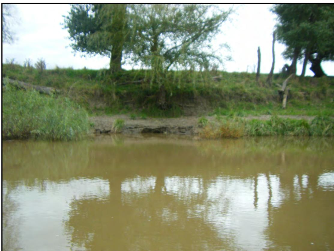
**Photograph 31:** Scour induced instability of bank located at upstream end of Section 6.
