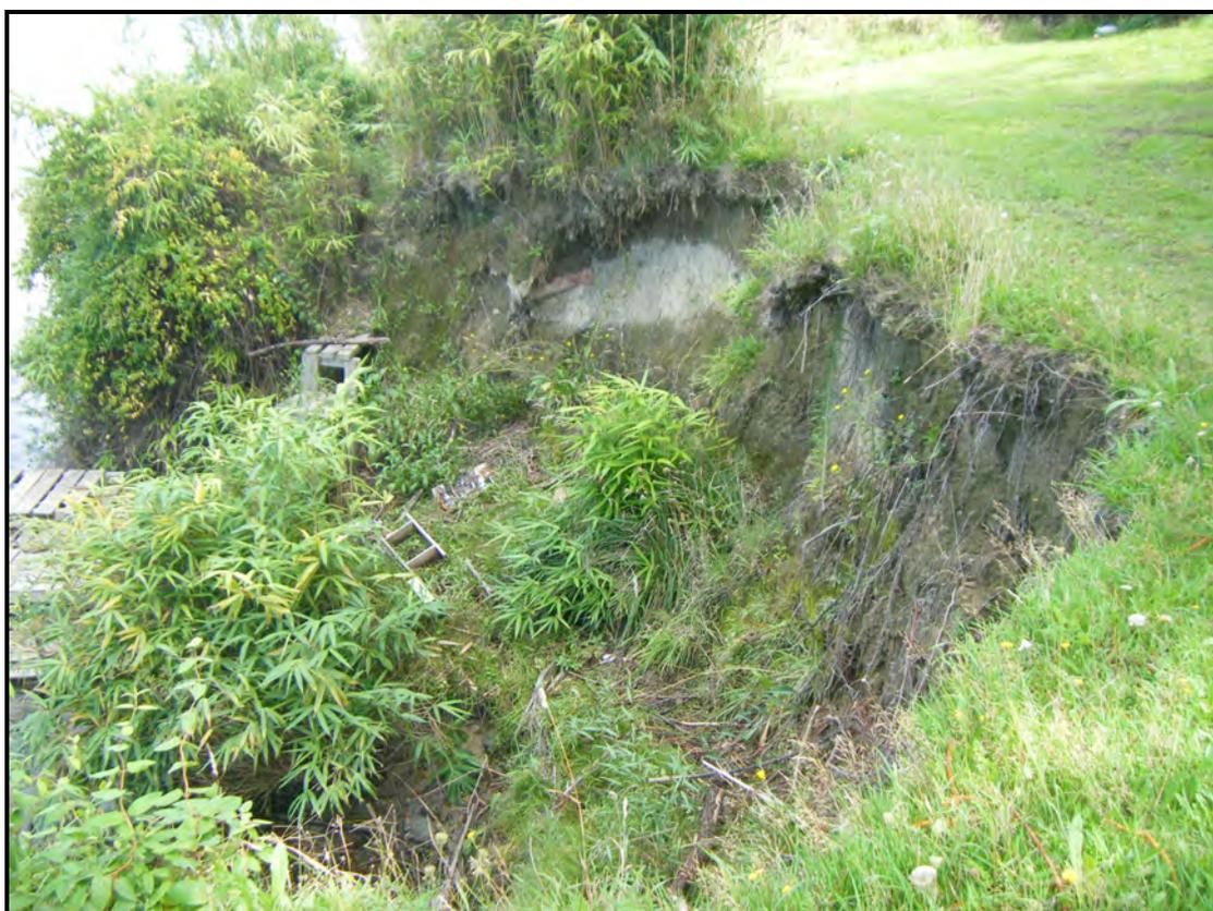
**Photograph 37:** Rotational failure of slope as shown from river in Photograph 35 above.
