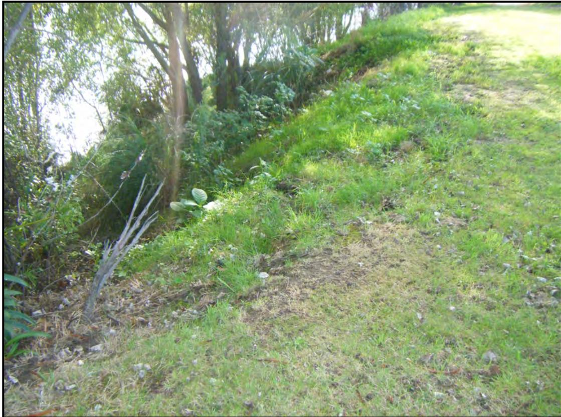
**Photograph 9:** Shallow instability of slopes at eastern end of Section 2.
