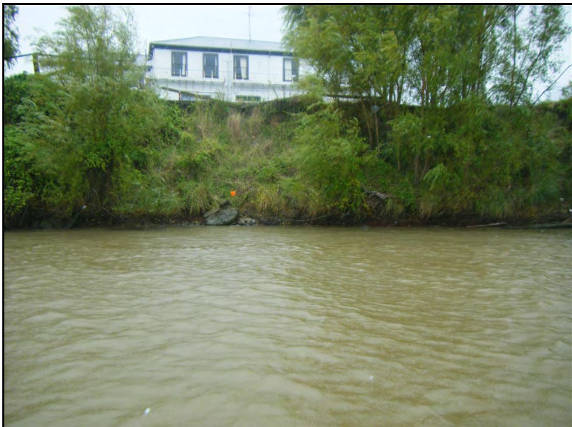
**Photograph 33:** Instability of heavily vegetated slope upstream of SH2 bridge adjacent to former motel.
