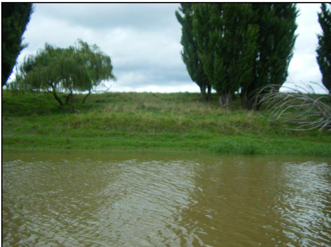
**Photograph 29:** Instability of lower sections of lightly vegetated slope in Section 6.
