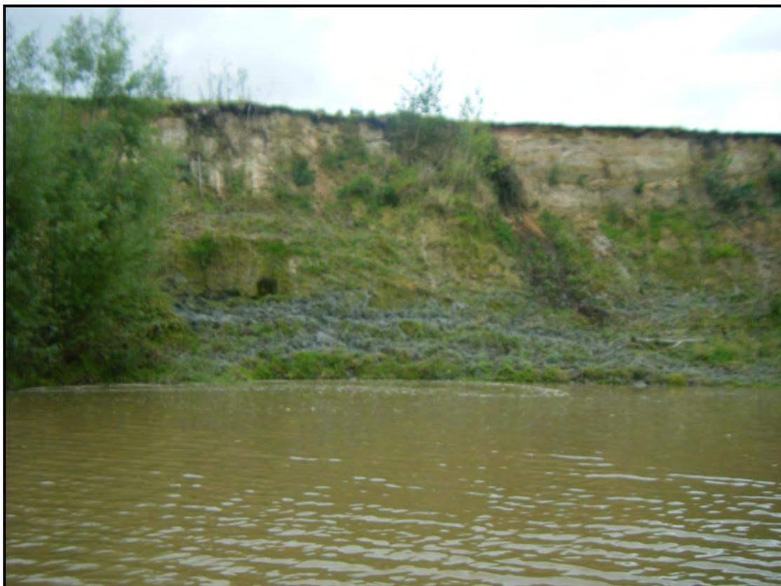
**Photograph 30:** Large scale instability of entire slope located within middle part of Section 6.
