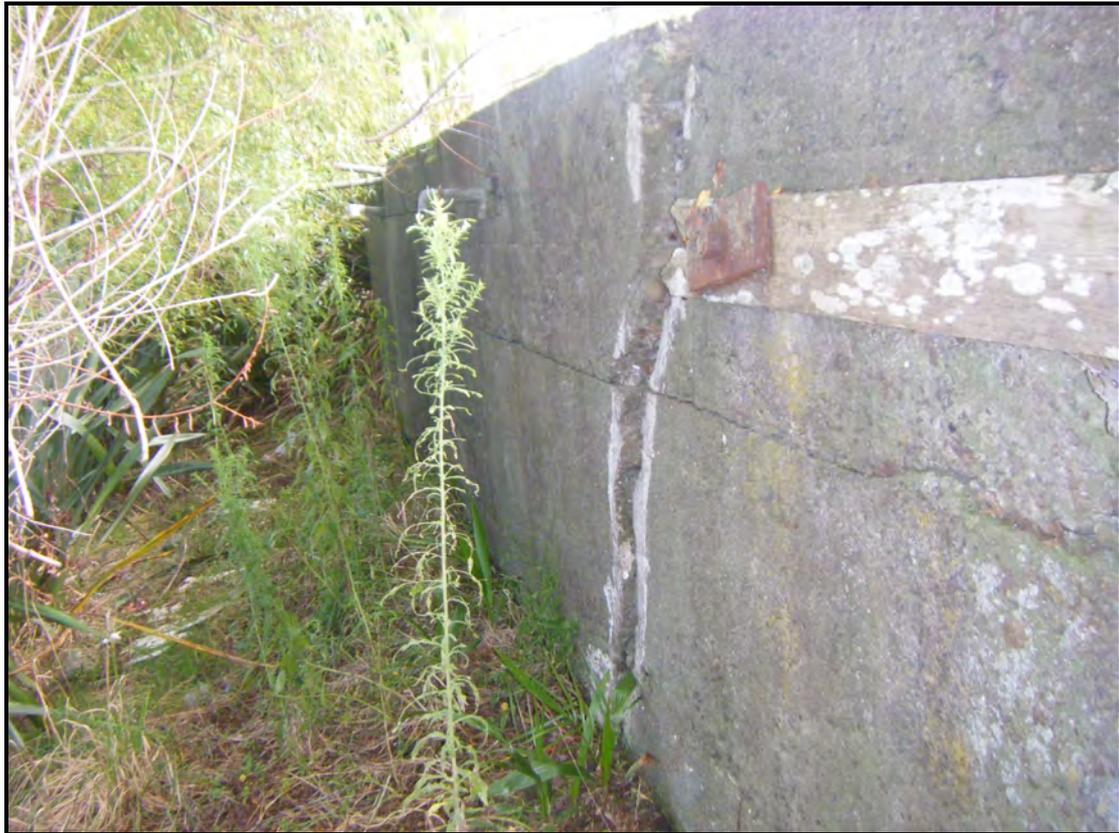
**Photograph 38:** Failure of concrete retaining wall adjacent to parking spaces on River Parade immediately upstream of SH2 bridge.
