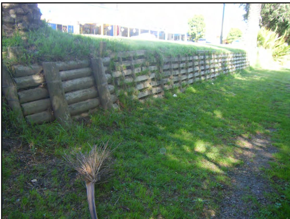
**Photograph 12:** 'Engineered' retaining wall on upper part of slope adjacent to Marine Parade close to Locke Street.
