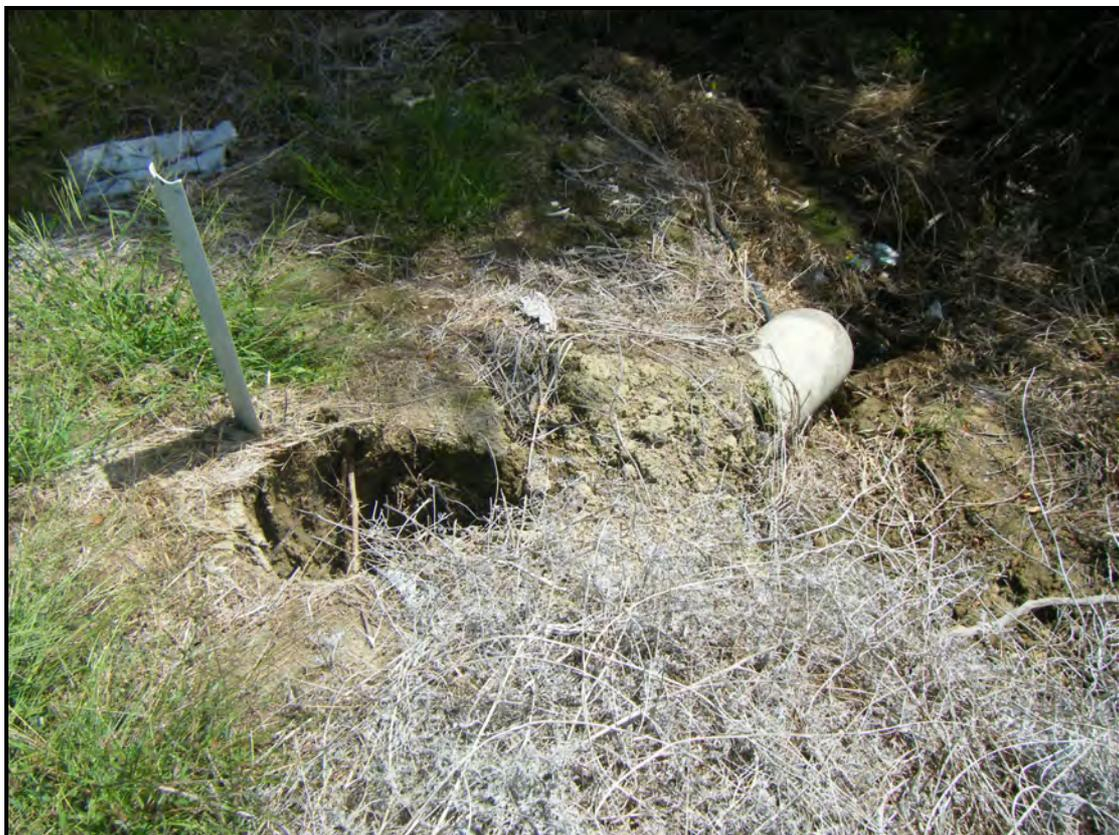
**Photograph 28:** Erosion and subsequent instability of slope adjacent to highway drainage outfall. Concrete pipe has collapsed and broken due to instability.
