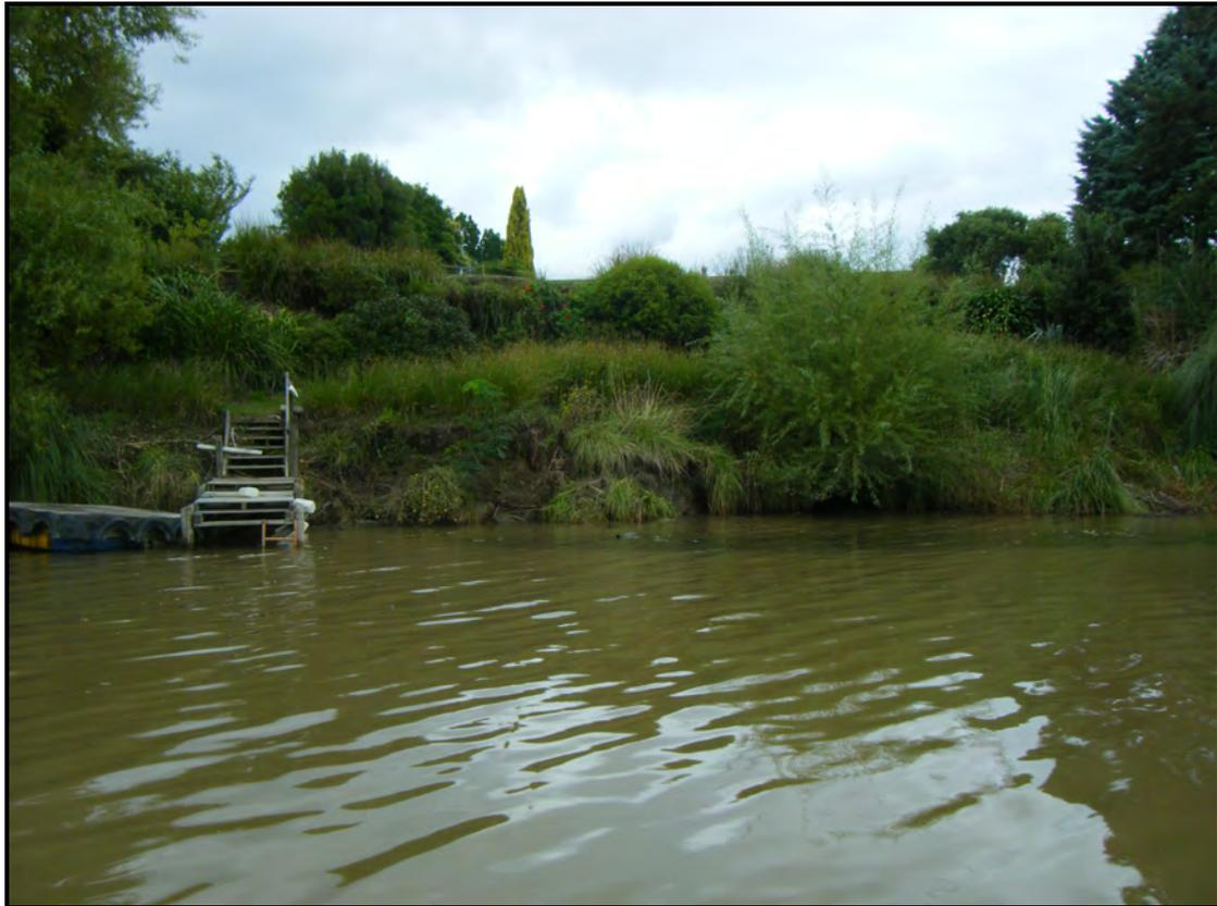
**Photograph 21:** Heavily vegetated slopes with signs of localised instability along right bank west of Churchill Street, at back of properties along Mitchell Road.
