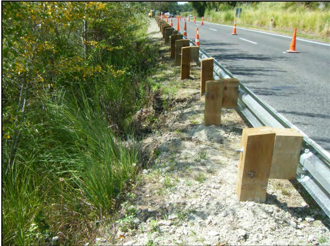
**Photograph 27:** Instability of upper part of 7 to 8m high slope adjacent to SH2 with new barrier recently completed.
